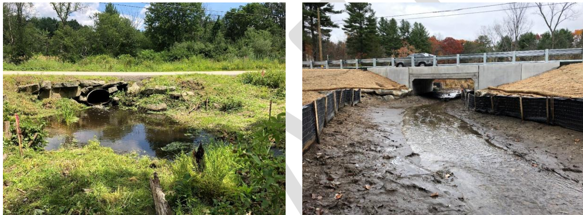
Figure 12. Culvert at Bay Road and Lubberland Creek in 2014 (left) and 2019 (right) (credit: TNC)
