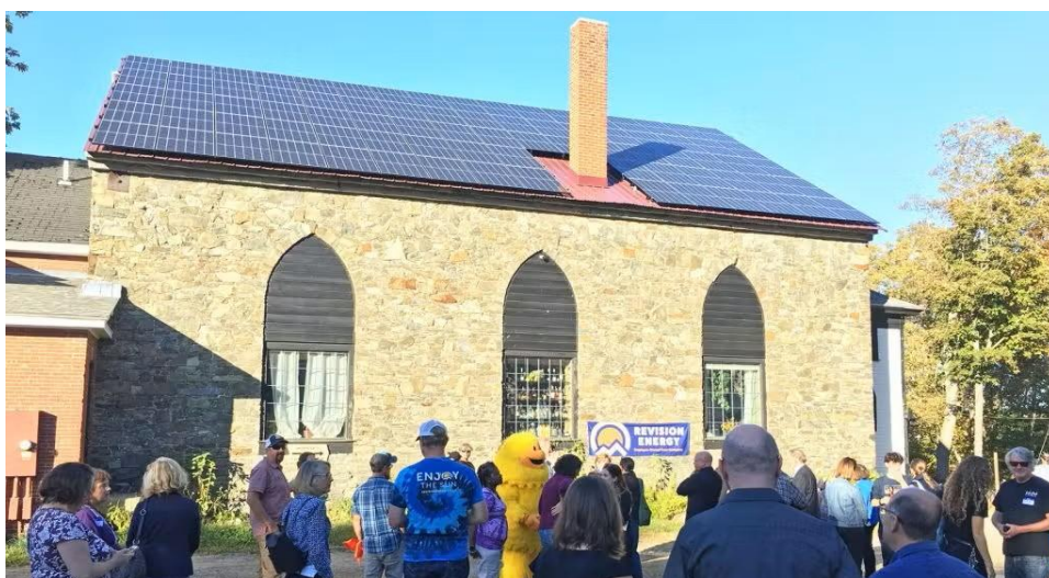
Figure 3 Stone Church Solar Panels (source: Revision Energy)
