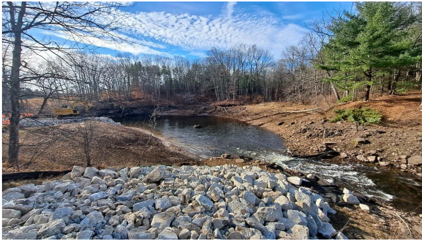
Figure 1 - Removal of the Gonic dam in November 2025 (SRPC)
