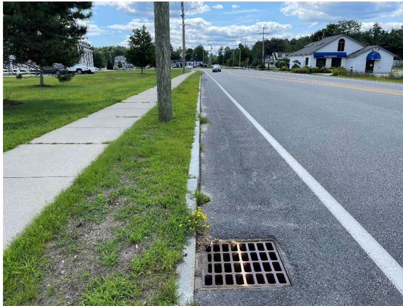
Figure 6 - Bike lane with grates on Route 108 near the Dover-Somersworth city line. Source: SRPC 2023.
