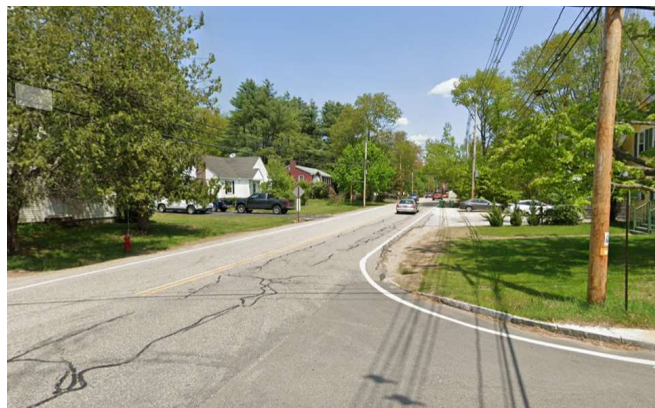
Figure 2 - Thanks to TAP funding, this section of Portland Street in Rochester will have an ADA-compliant sidewalk soon. Image source: Google (2023)
