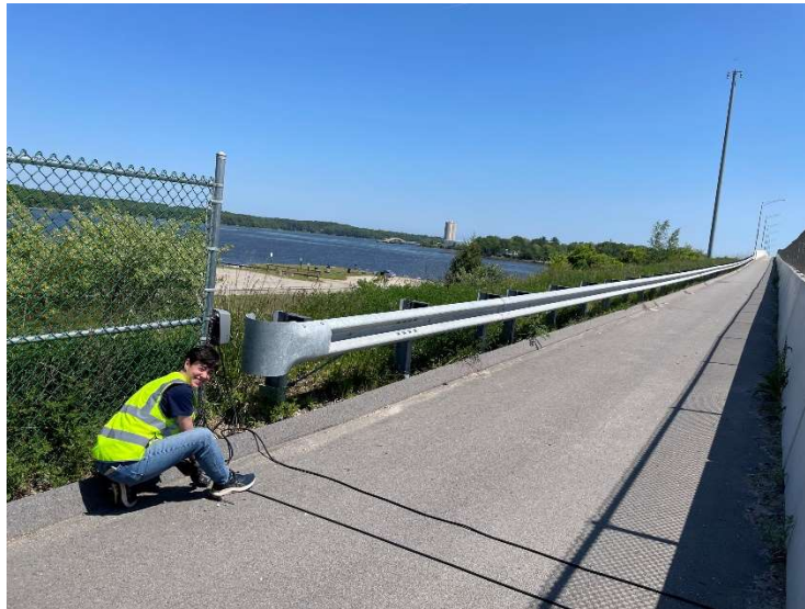
Figure 5 - 2023 Summer Intern Troy is seen installing tubing for the cyclist count on the Little Bay Bridge in June 2023. Source: SRPC 2023.
