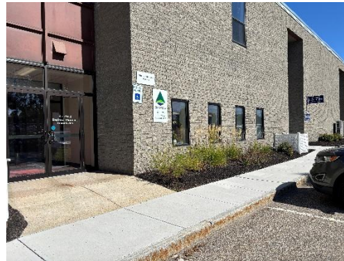
Main Office Entrance
